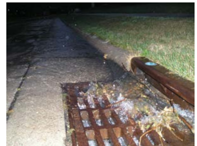
Stormwater rushing into a storm drain.
