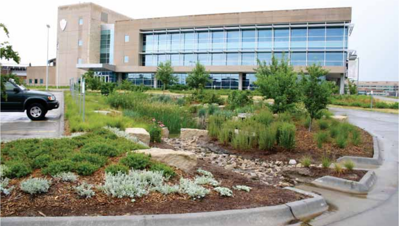
A stormwater detention cell near the front entrance of the Carl T. Curtis National Park Service Midwest Regional Headquarters, Omaha, NE, detains and filters water on this site adjacent to the Missouri River.
