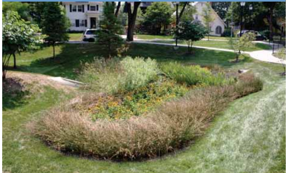
A rain garden constructed on a church site in Kansas City, MO, helps to filter and detain runoff from parking lot and street surfaces. The rain garden is part of the 10,000 Rain Gardens Program developed to help manage stormwater in Kansas City.
