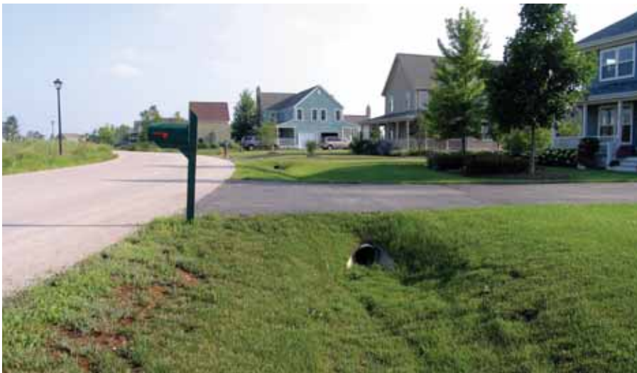
Vegetated swales have replaced traditional curb/gutter stormwater collection in conservation subdivision developments, like Prairie Crossing, Grayslake, IL, that have implemented successful stormwater management strategies.
