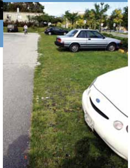
Vegetated paving surfaces allow water infiltration and generate cooler surface temperatures while providing a structural framework to support vehicle parking.
