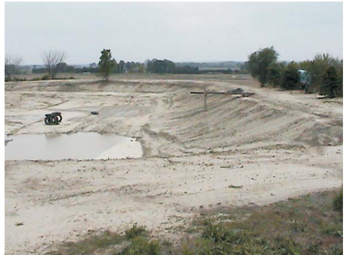
Wetland after construction
