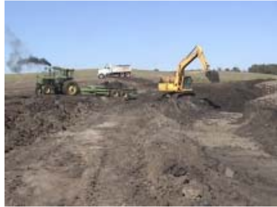
Solids were loaded into trucks and box spreaders.
