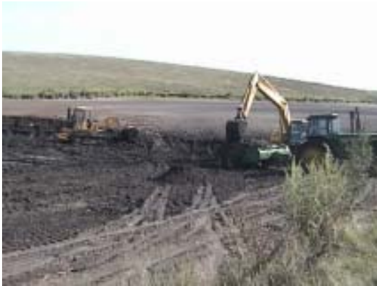
The average depth of excavation was 12 feet.
